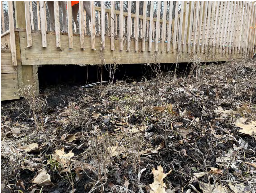
Photo 3 facing northwest: boardwalk clearance: permit application indicates construction of boardwalk with 4-feet of clearance to ensure underlying wetland would not be impacted.
