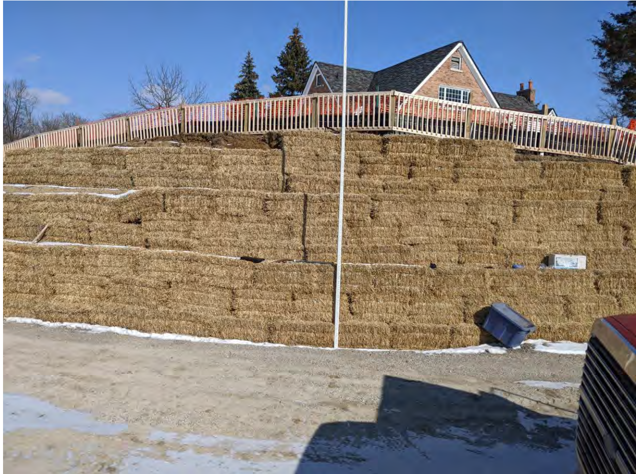
Existing 12-foot high excavation along property line.
