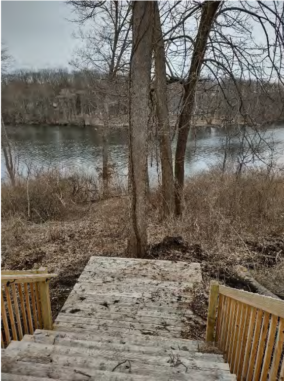
Photo 4 facing south: southern extent of boardwalk ends abruptly at base of tree. Mounds of soil and felled trees to the west of the landing.
