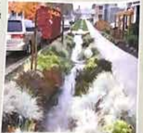
Sidewalk and bioswale in Seattle. Providing a bioswale between the path and road may eliminate the need for expensive curb and gutter treatments.
