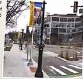
Curb protected bike lane on First Street in Ann Arbor. Note that in this configuration bike traffic is two-way within one lane, as opposed to one-way on either side of the street.
