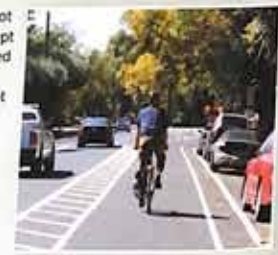
Dual buffered bike lane in Davis, California. The additional space to the right of the lane protects riders from unexpected car door openings.
