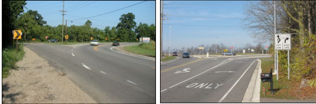
Photo 5-22: The Geddes Road/Superior Road intersection BEFORE (left) and AFTER reconstruction (right).
