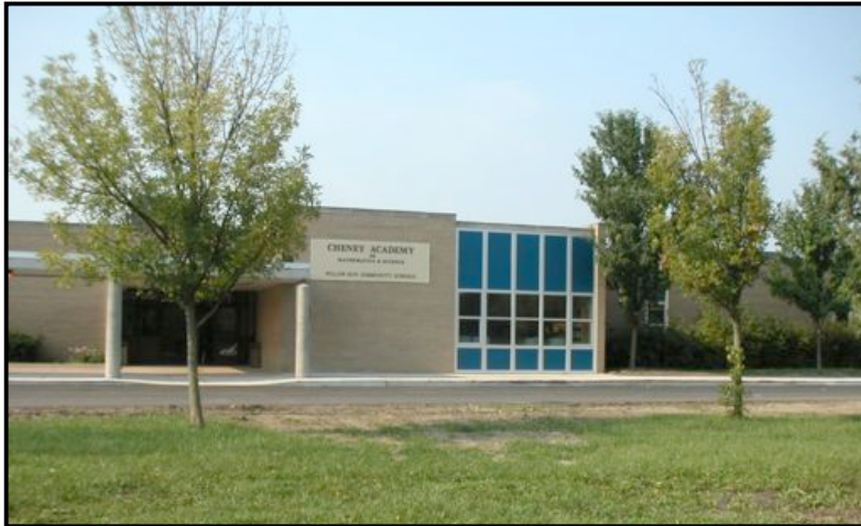
Photo 5-30: The Cheney Academy is one of the educational facilities serving Superior Township.
