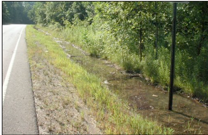
Photo 5-28: The stormwater drainage system needs to be carefully managed.
