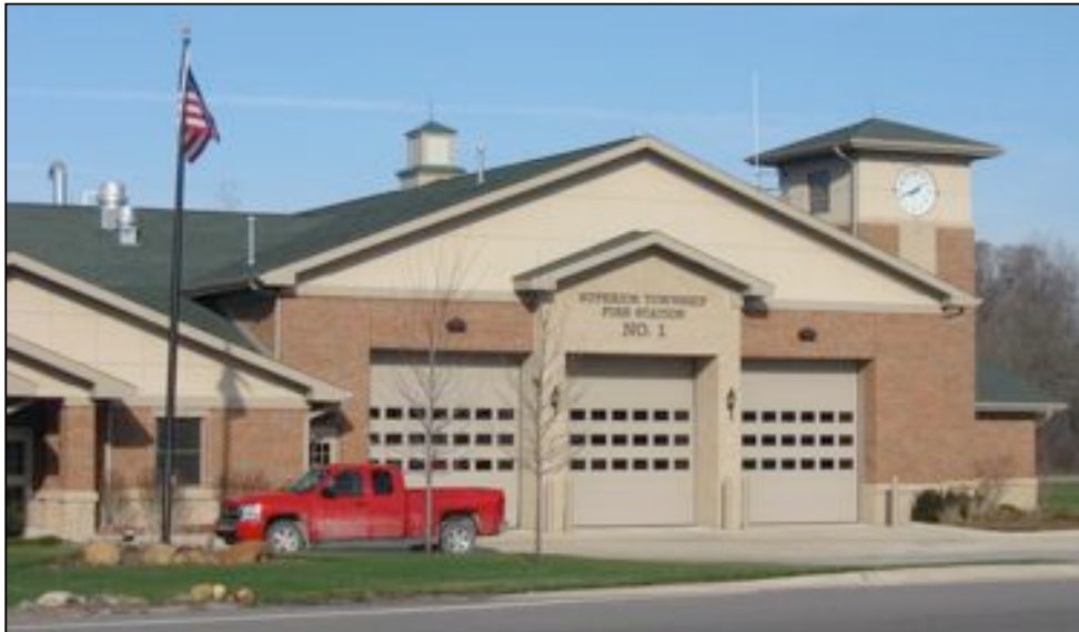
Photo 5-29: The Township's newest fire station is located at Ford Road and N. Prospect Road.
