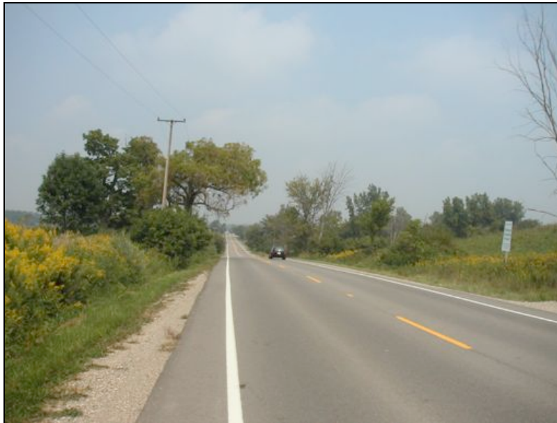
Photo 3-8: Rural roads in Superior Township include both paved and gravel roads.
