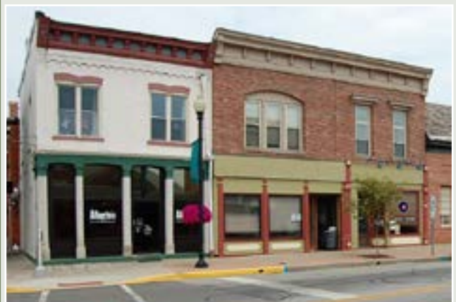
Second story apartments in commercial buildings provide additional housing options within the context of neighborhood commercial use.
