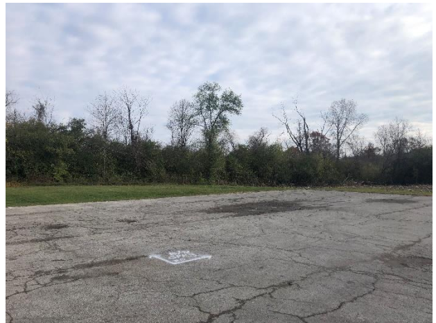
Picture 2: This photo shows the site from the SW corner. Scan boundaries were marked in the field.
