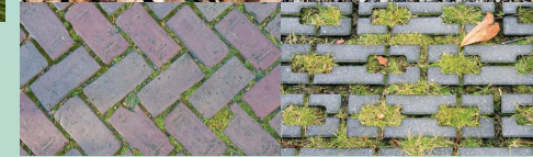
PERMEABLE PARKING LOT PAVING OPTIONS
