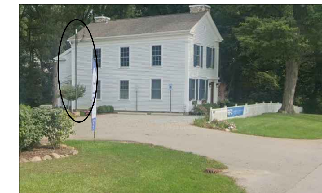
SIMILAR PARKING LOT LIGHTING IN NEIGHBORHOOD AT 5263 PLYMOUTH ANN ARBOR ROAD
