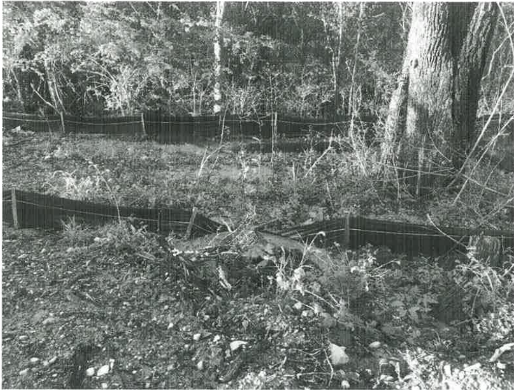
Photo 1: Silt fence failure at bottom of slope
