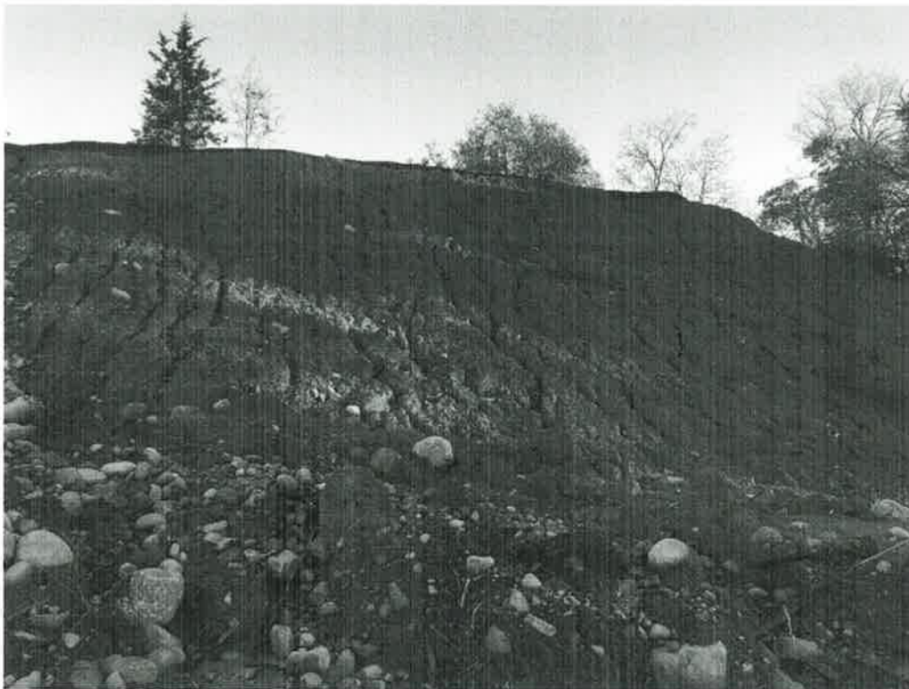
Photo 2: Erosion along slope (typical)
