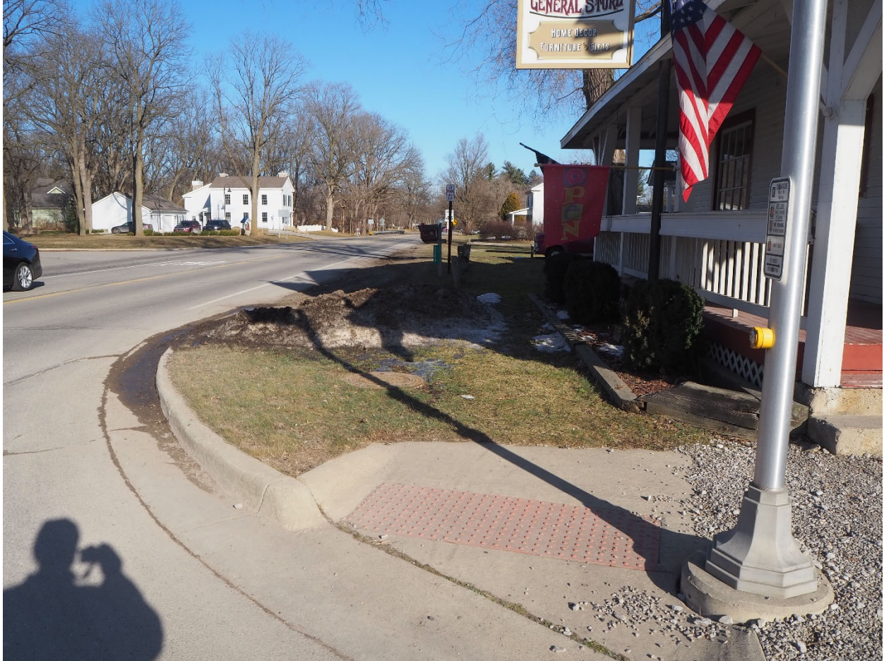
Southeast corner of Plymouth Road & Cherry Hill Road. Looking east. Existing sidewalk in front of address 5206 Plymouth Road.
